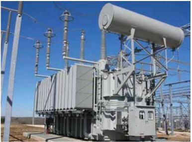
In addition several diagnostic features can be in built into the systems that are helpful in the transformer asset management. These can cover transformer loss of life, tap statistics, real time over load capabilities etc. The system is capable of interfacing with several third parties individual IEDs such as Dissolved Gas analyzers, Bushing monitors, Fiber optic hot spot measurement systems, Smart breathers etc.
